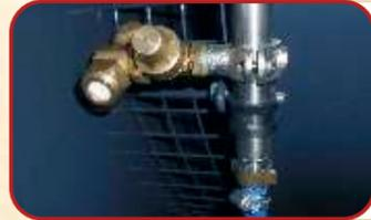
Stainless steel hold-nozzles and double brass nozzles with check valve
